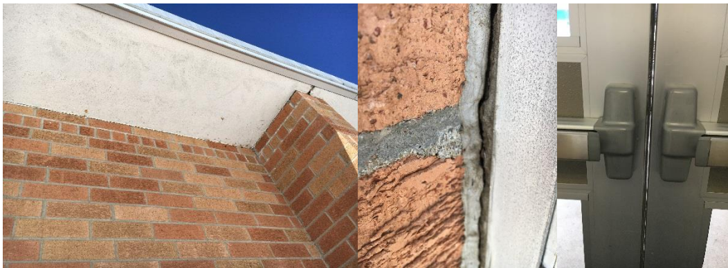
Figure 8 - Building Envelope Deficiencies
