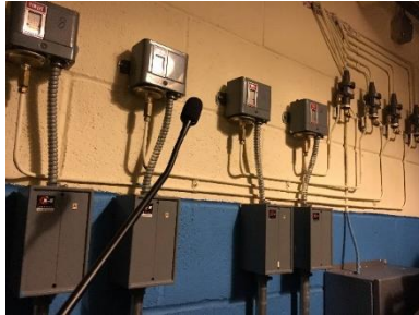
Figure 15 - Pneumatic Control System
